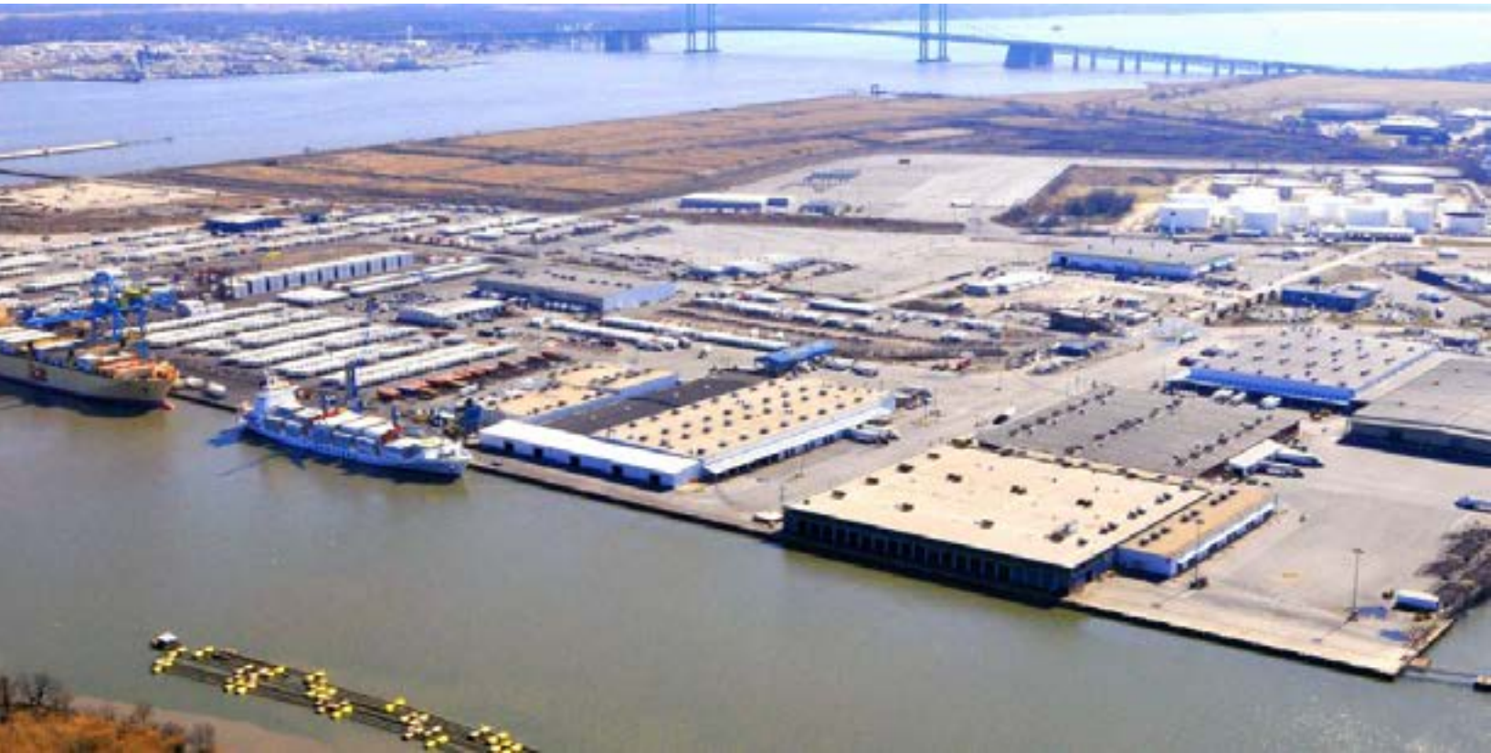
Port of Wilmington, Delaware. Photo Credit: portofwilmington.com.
